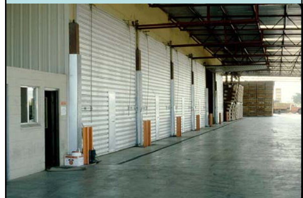
Citrus Degreening Rooms
