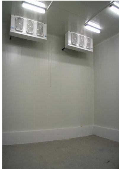
Gastight floor (concrete)
